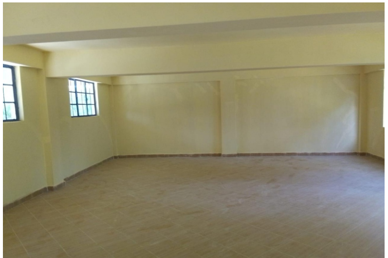
Construction of 8 No. Classroom Block at St. Cecilia Olare Primary School
